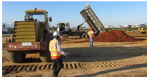
Importing fill material for the pile structure foundation (Photo: CDM Smith)
