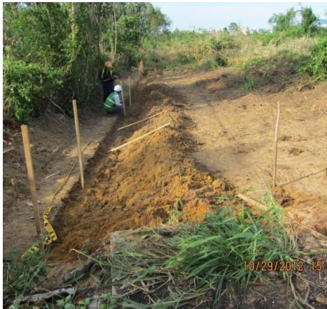
Installation of Silt Fencing (Photo: CDM Smith)
