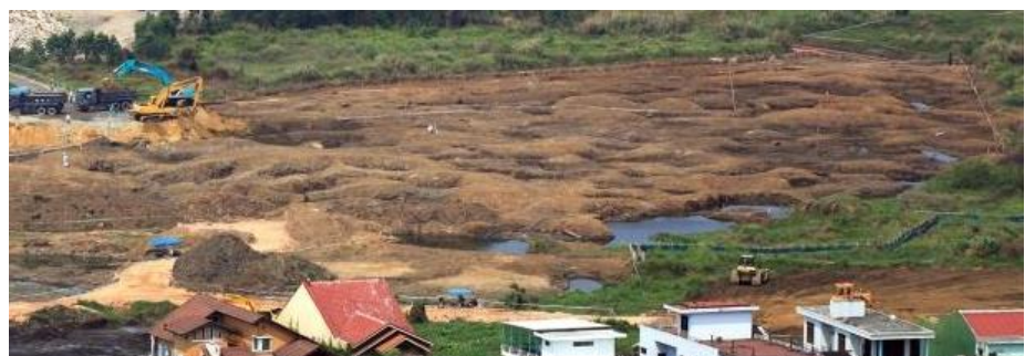
Excavation in the wetland area
