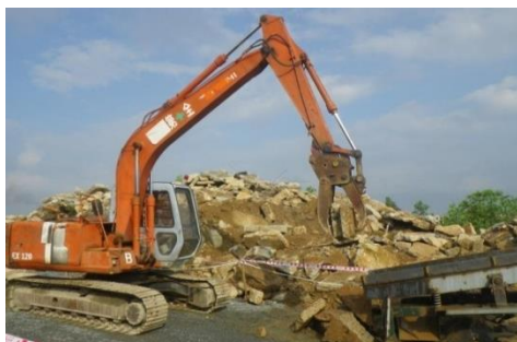
Cleaning and preparing concrete for crushing
