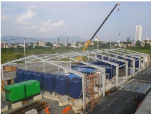
Liquid/vapor treatment plant construction
